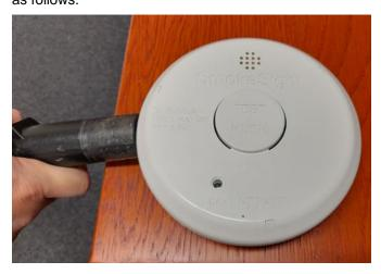
Remove the SmokeSight alarm, remove the batteries, place in a dust free plastic bag and return to Redbusbar for reprogramming. The ceiling mounted base can remain installed.
